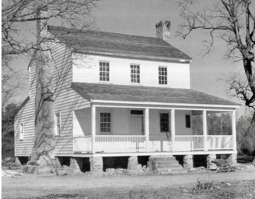
Farmhouse. Walnut Grove Plantation, 1765, SC, is a classic, Southern I-House, a simple, symmetrical clapboard house with attached porches. The style was so popular that it migrated well beyond the South, eventually becoming the iconic American farmhouse from coast to coast.
