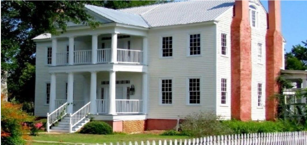
Federal. Palladian inspired double portico with taller Greek orders supporting at the lower porch create a sense of proportion to the shorter columns at the upper porch, note Palladian window in the side
