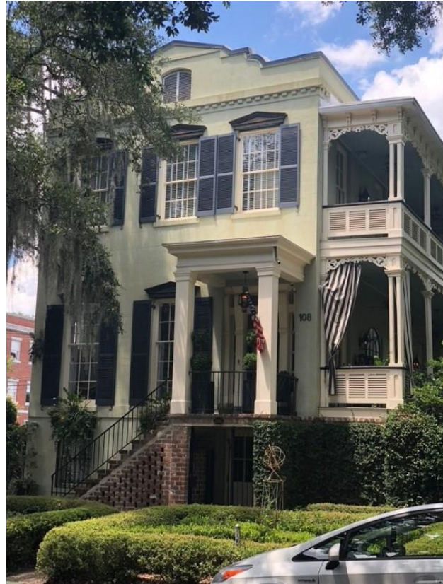
Savannah Town House. 108 Jones Street, Savannah, GA; Greek Revival pediments over windows; piazzas could have been modified or added later given the Victorian detailing at the cornice.
