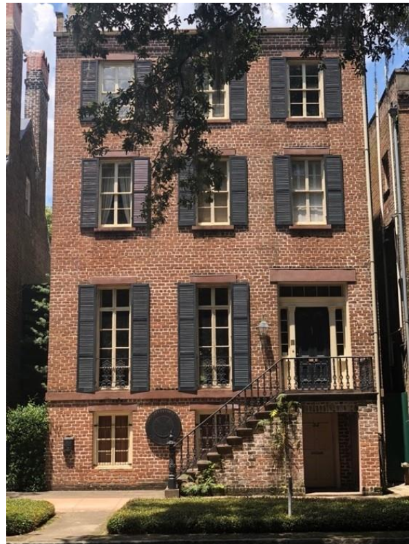
22 Jones Street, Savannah; simple stone or cast stone lintels over every door and window.
