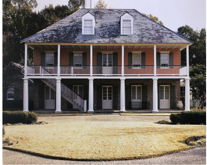
French Colonial with exterior stair adjoining porches, an example of the changing refinement with Greek Revival influences by the use of the Tuscan Columns on the first floor.
