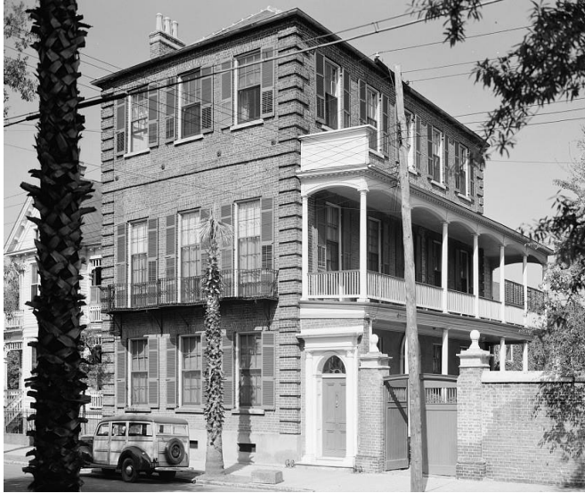
Charleston Single House. Thomas Heyward House, 18 Meeting Street, Charleston, SC. Note: Taller windows on the more prominent second floor, also known as the Piano Nobile.
