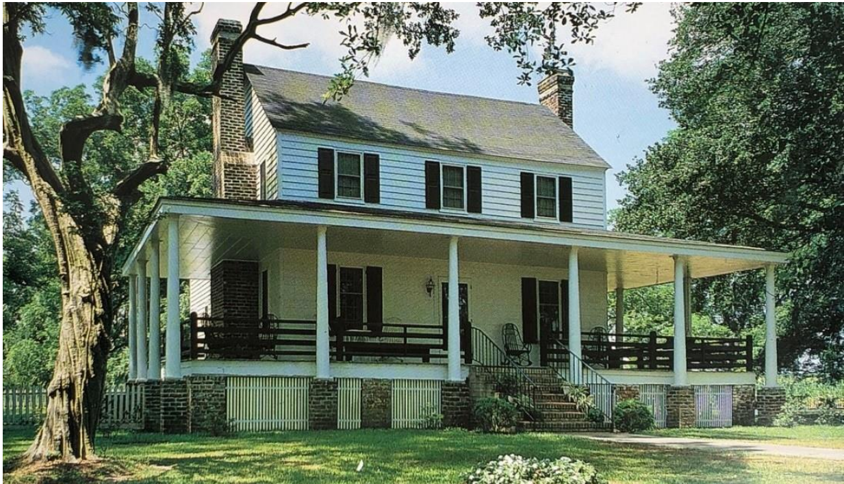
Farmhouse. McGill House, 1767, Prince Frederick's Parish, South Carolina. Special note: columns stand free of the balustrade and chimneys at the second floor stand free from the house to avoid necessary flashing.
