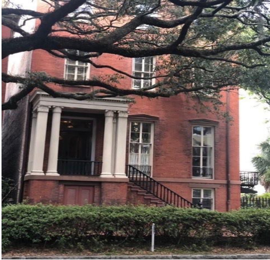
Savannah Town Houses. Example of a classic Savannah Town House: 10 West Jones Street, Savannah, GA. Town house with a covered stoop and iron railings (originally wood). Tall casement windows on the second floor, made to look like double hung sashes. Cast stone pediments adorn the tops of these elegant windows. Note the typical raised basement.
