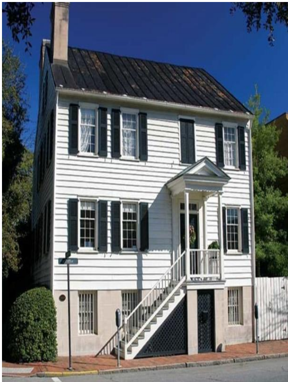
Savannah Town House. Federal style town house, raised on a full basement, Francis Stone House, Savannah, circa 1820.
